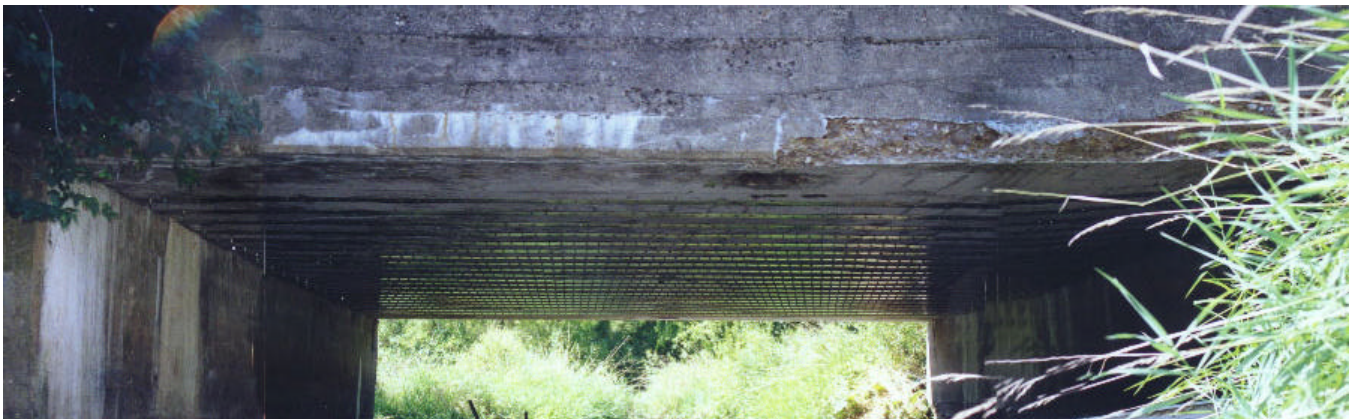
Figure 3. Retrofit of Edgerton Bridge using Power Actuated System.
